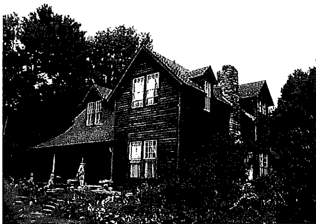
In December of 2002 the owners of the Vardell House (also known as Opicherhoka) in Blowing Rock placed an easement on the house and its surrounding 1.76 acres to ensure its protection in perpetuity. The easement protects the historic features of the home and prohibits subdivision of the land to ensure its serene setting for generations to come.
