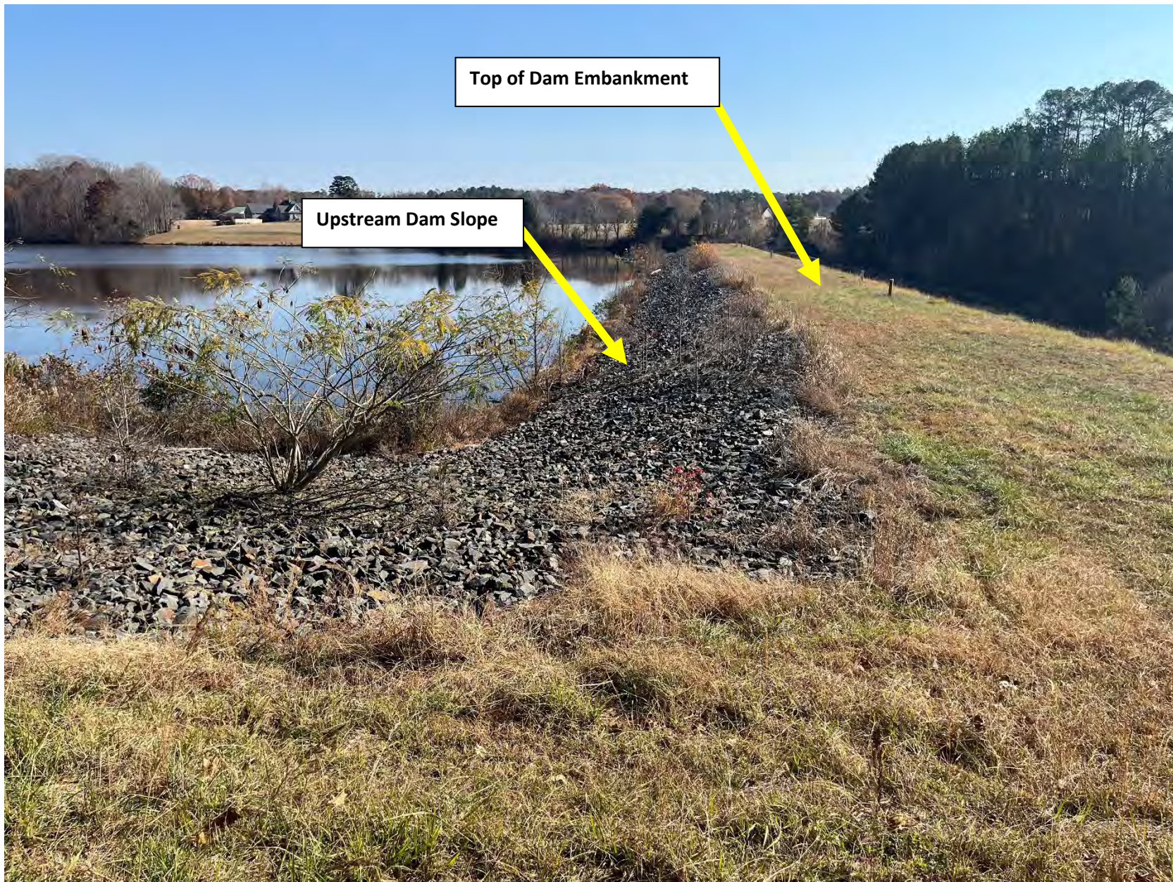
SITE PHOTOS: Black Run Creek Dam
