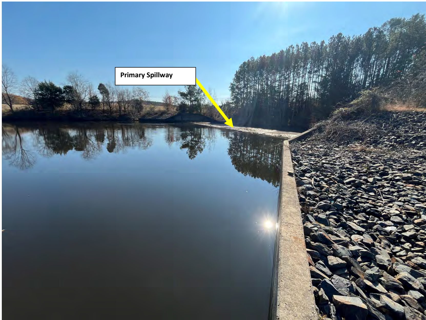
SITE PHOTOS: Black Run Creek Dam
