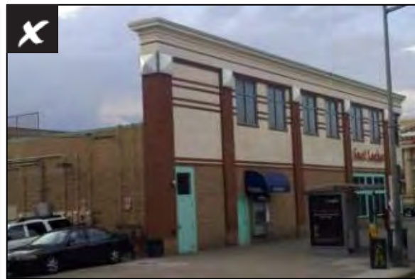
Non-continuous false front parapet without height changes
