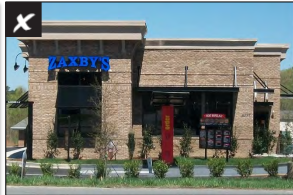
Drive-through ordering station on front facade
