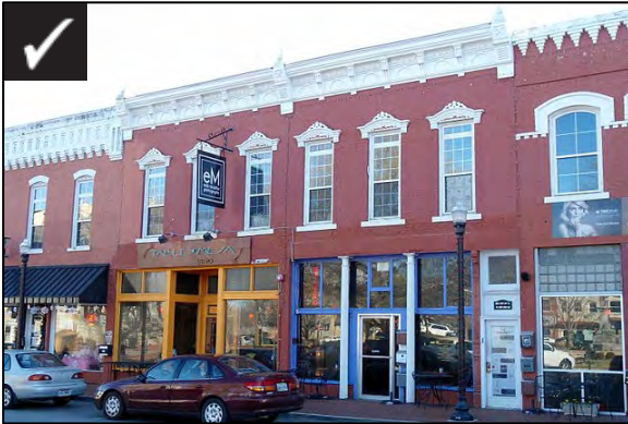
Brick façade with bright accents
