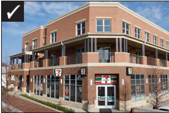
Brick façade with formed concrete accents
