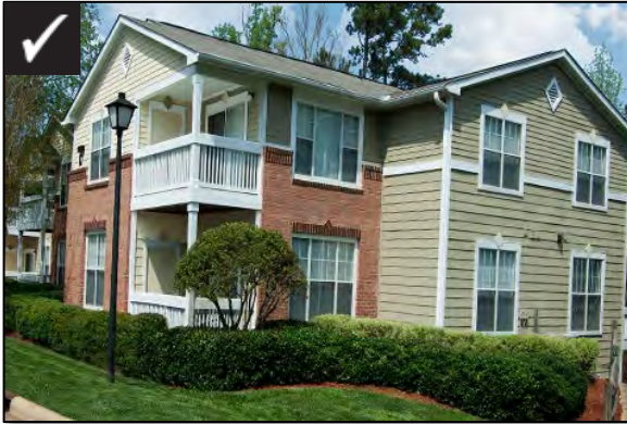
Adequate windows with regular rhythm and alignment
