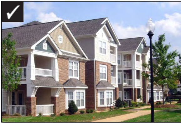
Proportional roof with variation and overhang
