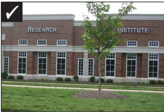
Continuous parapet with height changes
