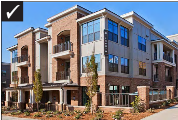
Flat roof with decorative parapet and variation
