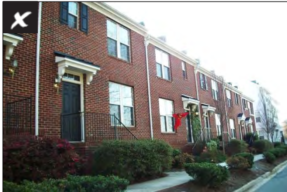
No façade articulation
