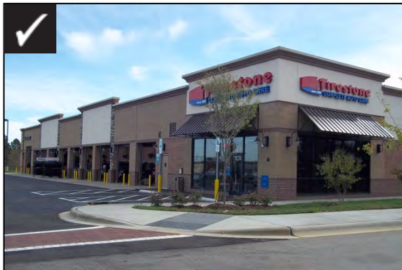
Service bays on secondary building wall
