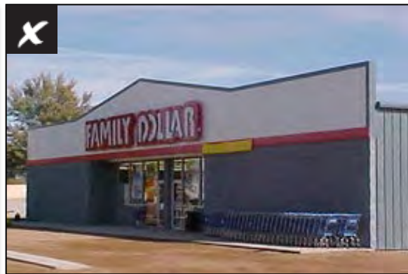
Painted concrete block and metal facades
