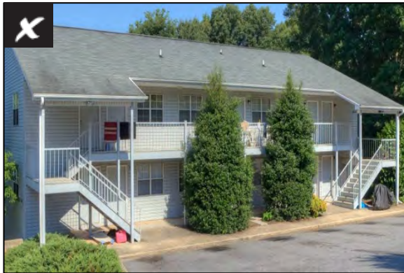
Exterior stairs and circulation corridors
