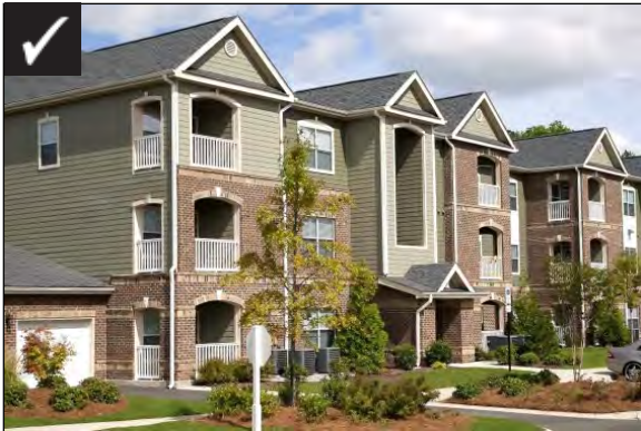
Façade articulation with recesses and projections
