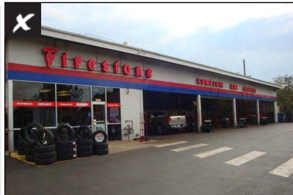
Service bays on primary building wall
